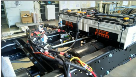
Power Distribution Board Main fuse box (1X 150A)
